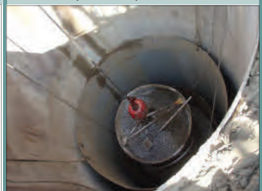
Placing aggregate fill around barrel
