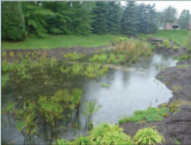
Stormwater ponded in the bioinfiltration basin during a rain event.
