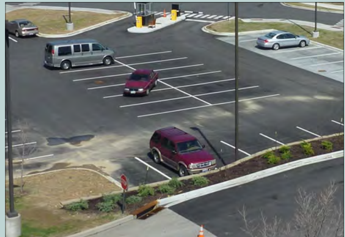
Excess silt and sediment on the porous pavement surface can prematurely clog the system.
