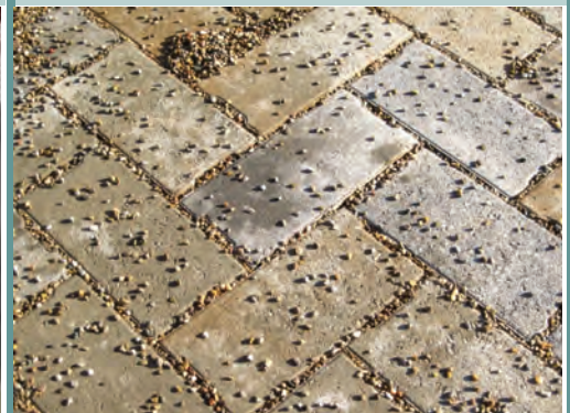
Permeable Paver Aggregate Installation
