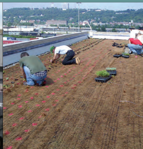
Planting through temporary wind blanket
