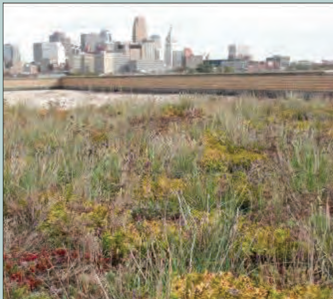
Extensive vegetative roof at Cincinnati Museum Center.
