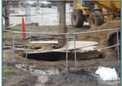
Drilling drywell with auger
