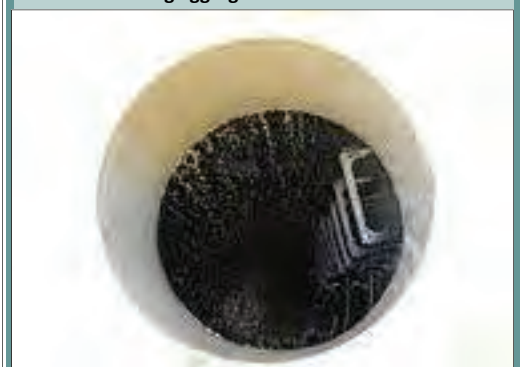
Completed drywell without casting
