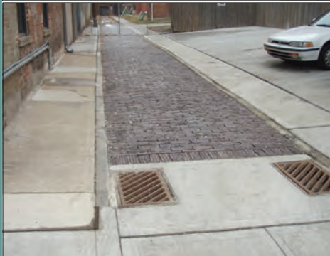
Osborn Alley Construction
