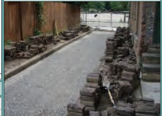
Comer Alley Construction
