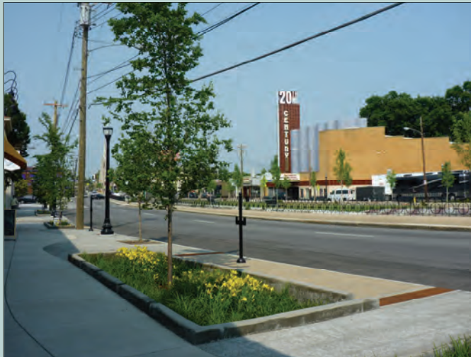
Bioretention planter box.
