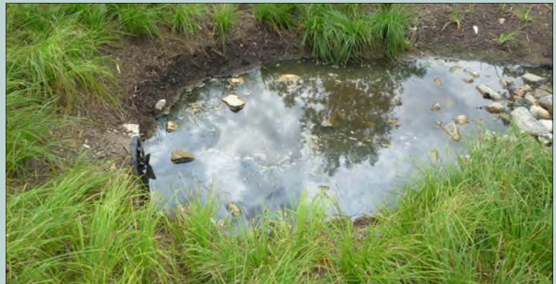
Water ponded in this forebay caused stagnation and conditions amenable for mosquito breeding.
