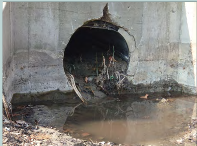
Debris and foreign material from an existing pipe draining into a retrofitted detention basin.
