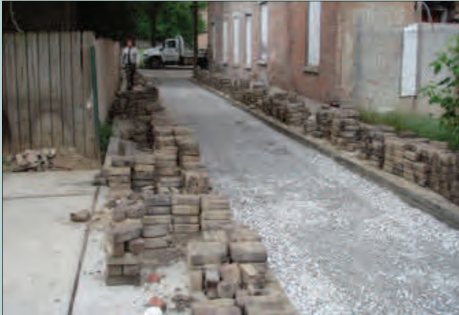
Existing pavers prepared to be reused as a porous pavement system.
