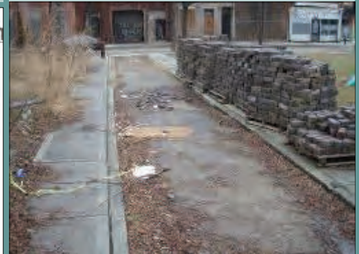
Comer Alley Construction
