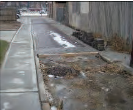
Osborn Alley Construction
