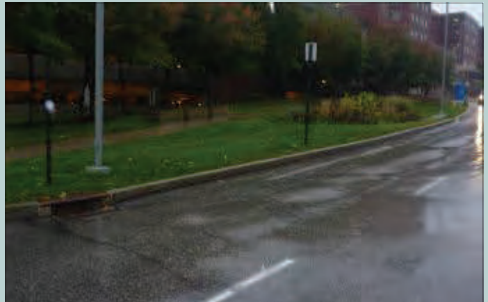
Stormwater runoff enters the combined sewer system.
