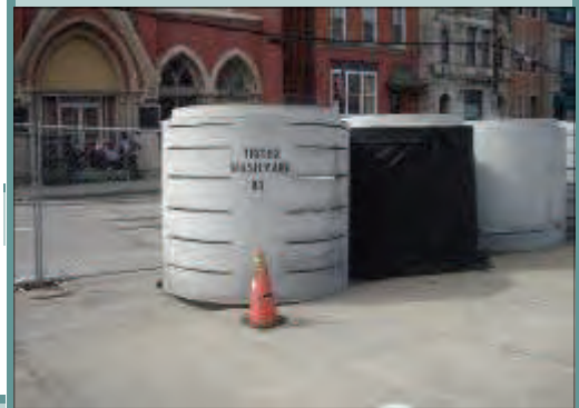
Drywell barrels pre-installation
