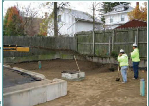
Installation of Engineered Soil
