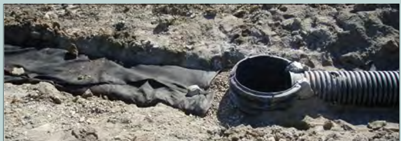
Filter fabric and an underdrain being installed.
