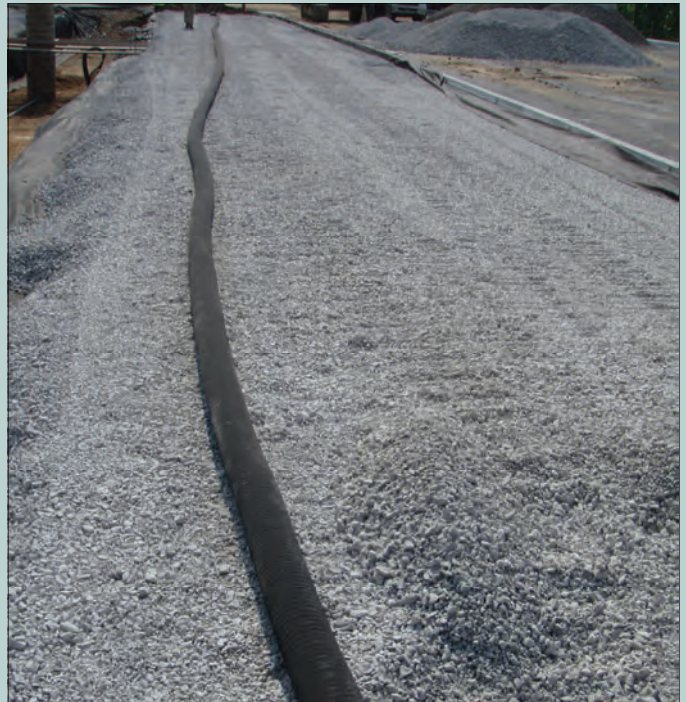
Underdrain to be installed in the bioswale.
