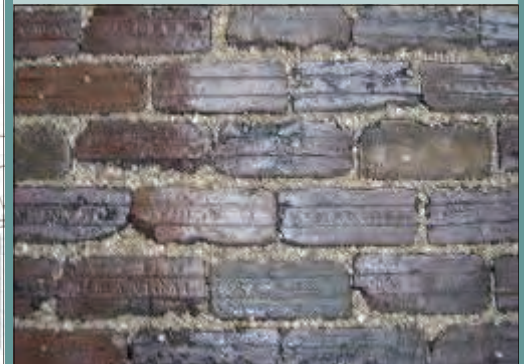
Comer Alley Permeable Pavers
