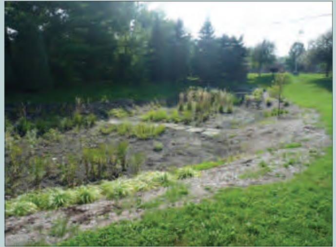
The stormwater has infiltrated through the system 24 hours after the rain event.
