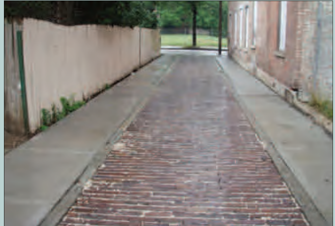
Newly installed porous paver alley.
