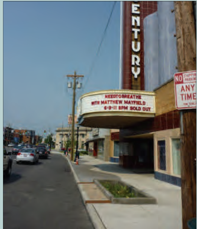
Stormwater planter located outside entrance/exit to theater.
