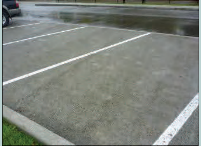
Porous concrete at Hartwell Elementary.
