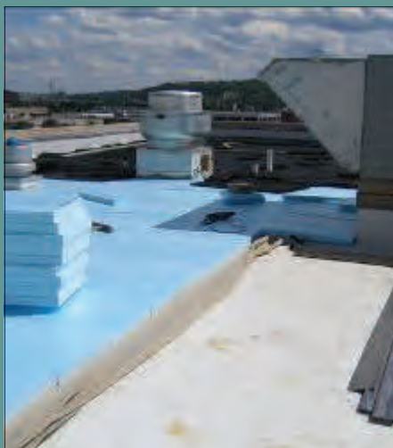
Roof membrane, fabric, and insulation
