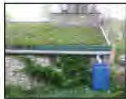
Fig. 1. Sloped green roof at Civic Garden Center of Greater Cincinnati, used for monitoring of runoff water quality on full-scale roof.
