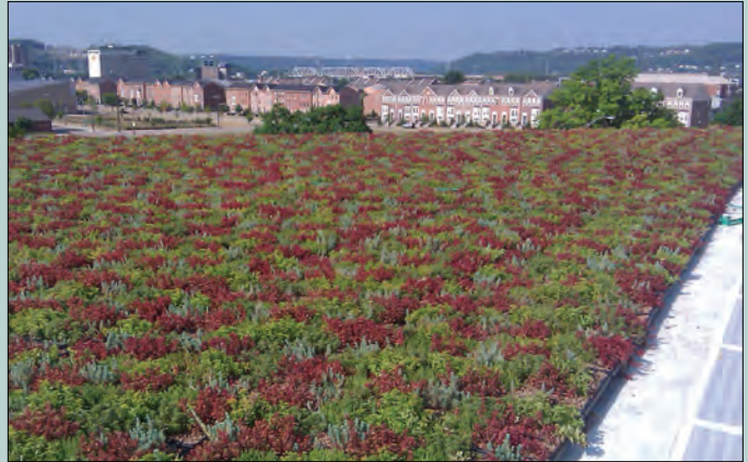
Extensive vegetative roof at Taft IT High School.
